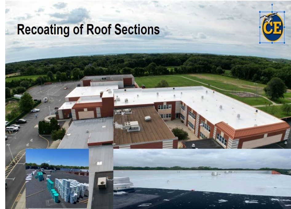
Completed roof sealcoating at elementary school
